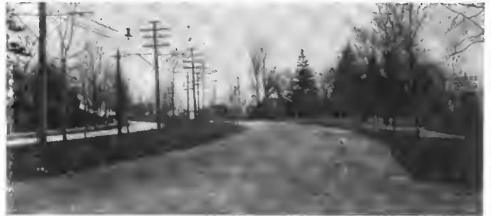
SECTION OF NEWTON BOULEVARD TREATED WITH TARVIA.
